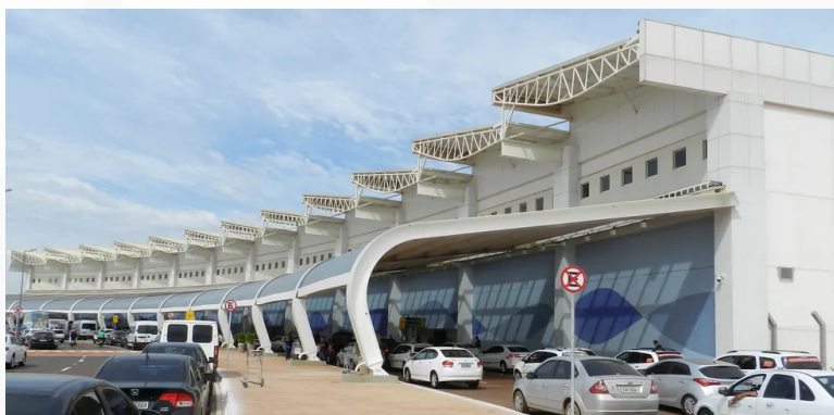
Santa Genoveva Airport in Goiânia/GO. Source: Infraero/ Disclosure
